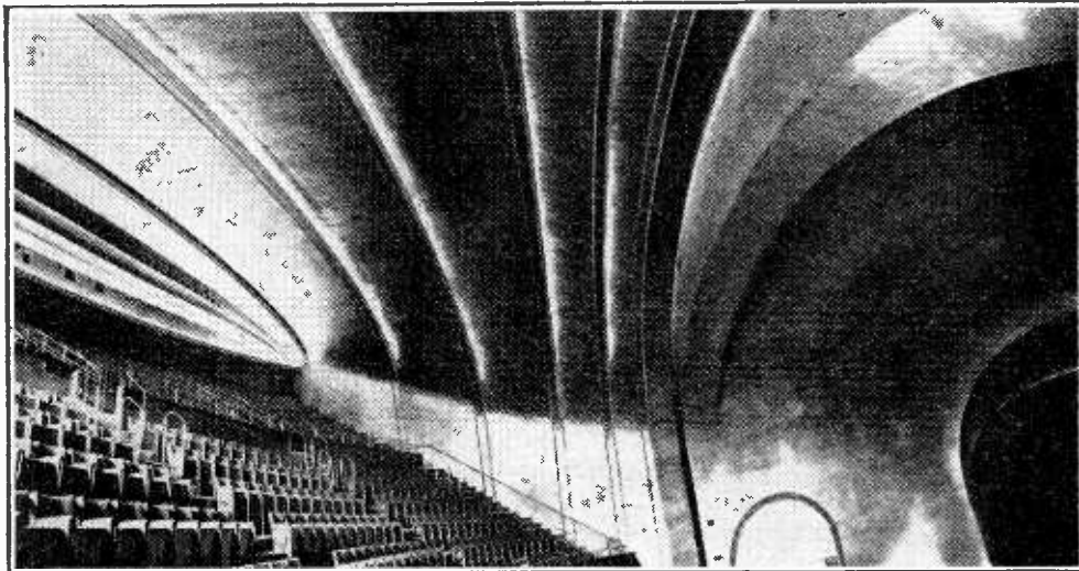
The ceiling of the Cambridge Theatre, Gt. Earl Street, London, W.C.2, is designed in accordance with the principle illustrated in Fig. 4.
